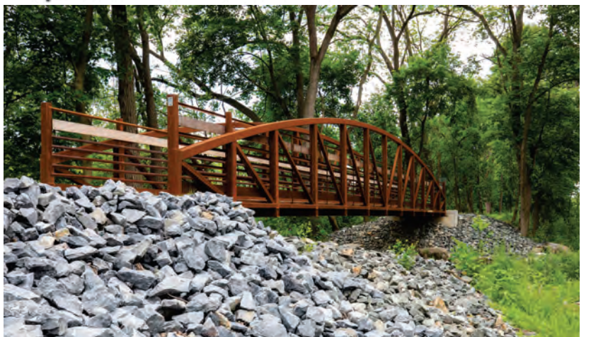
Contech Capstone style pedestrian bridge
